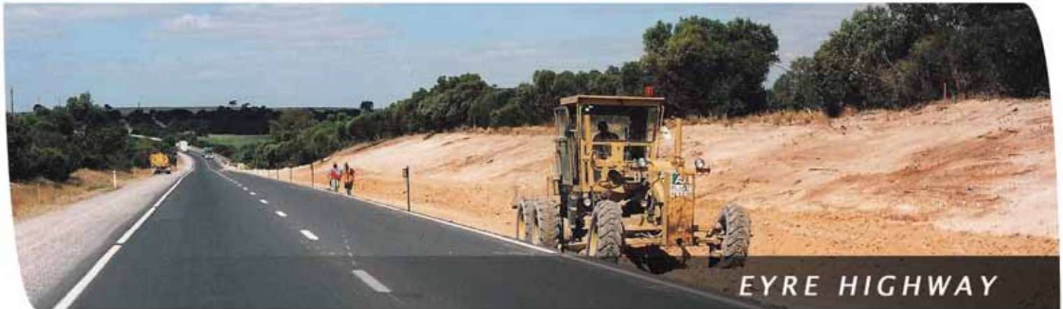
A grader levels the work area
